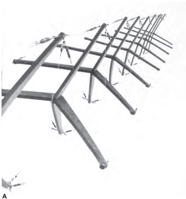
• Fig. A1.76 (A) More complex tensegrity structures like this mast begin to echo the spine or rib cage. (B) Designer R. Buckminster Fuller with a geometric model. (Reproduced with kind permission from the Buckminster Fuller Institute.)
