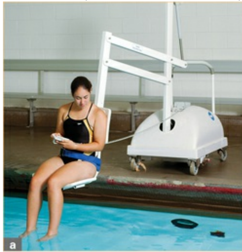
Figure 25.3 (a) Lifts are a primary means of access according to the ADA guidelines. (b) Gradual-slope entry is a primary means of access. (c) A dry ramp provides access to a transfer ledge. (d) A transfer system can be a secondary means of access.
